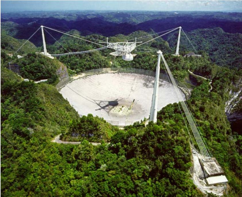
Figure 1.7. The Arecibo radio telescope; 305 meters in diameter. The platform suspended above the reflector weighs 500 tons (photo courtesy of the NAIC – Arecibo Observatory, a facility of the NSF).
